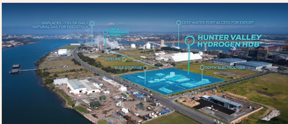
The Hunter Valley Hydrogen Hub at Kooragang Island, New South Wales. Photo courtesy of Orica.
