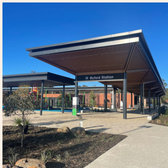
Byford Railway Station in Perth, Western Australia. Photo courtesy of Public Transport Authority of Western Australia.
